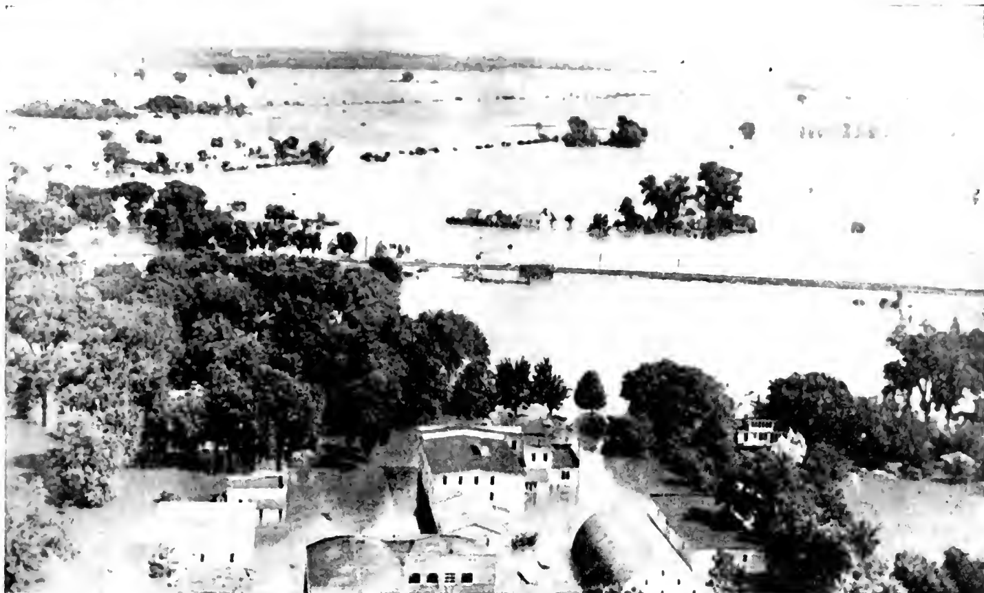
Downstream—recurring floods inundate millions of acres, waste water, topsoil and latent energy, damage farms, roads and cities
